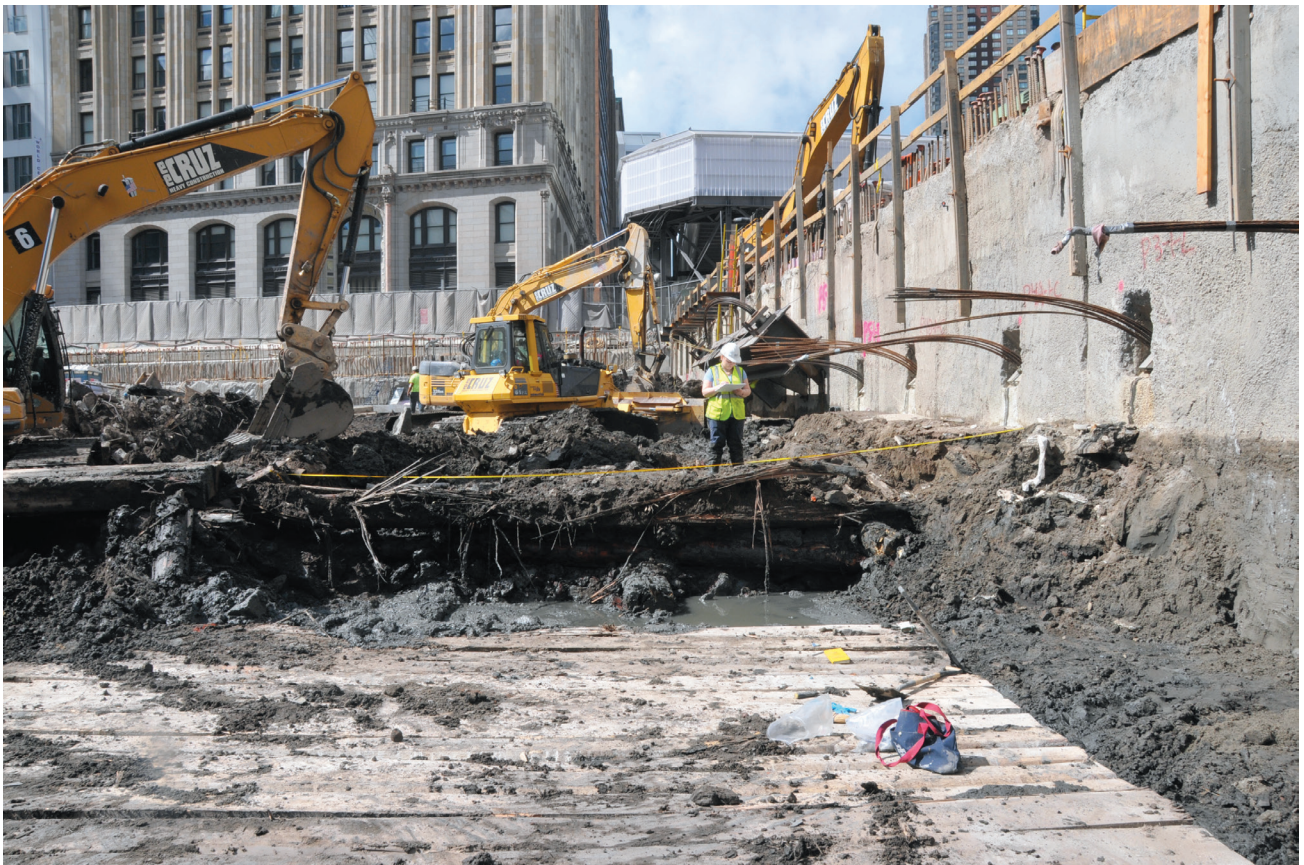
Photograph of 2010 monitoring during excavation of the World Trade Center Vehicular Security Center Project. Photograph by AKRF, courtesy of LMDC.
